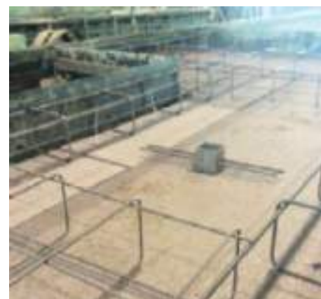
Isolante posato Insulation installed
